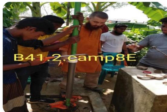
Tube-well repair at Camp-8
